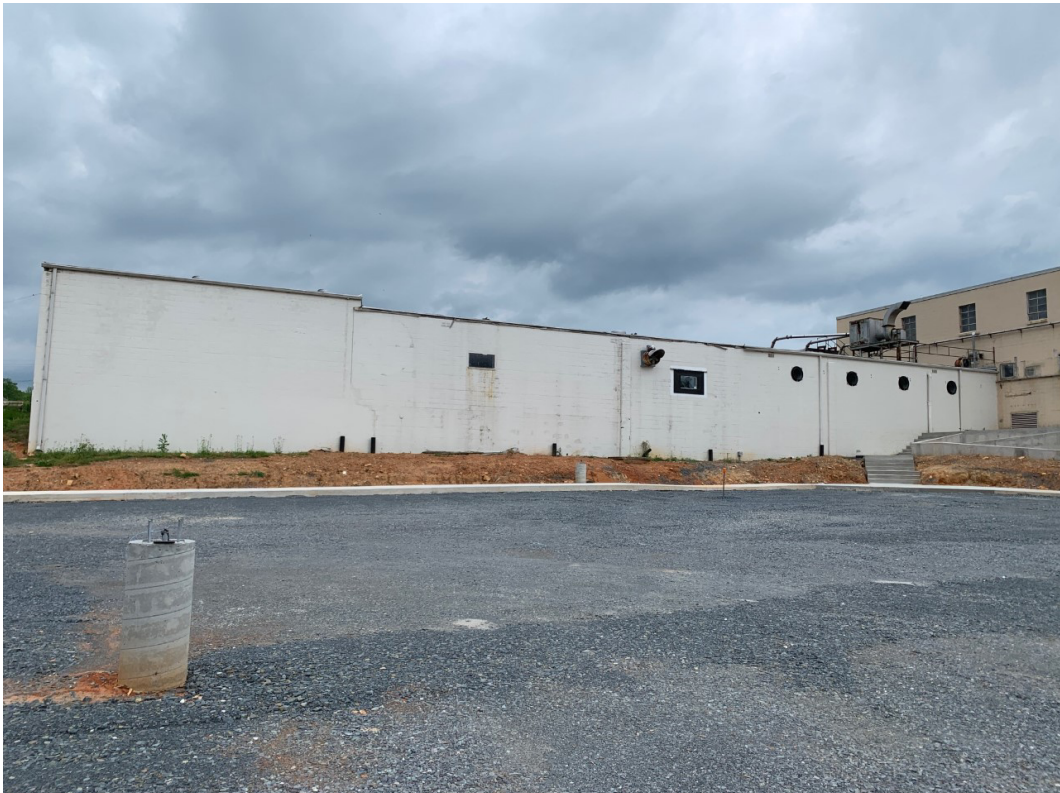
Site # 2, wall facing future main parking and entry area – 10' x 25'
